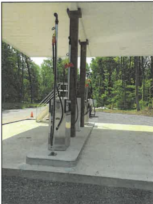
Fuel Dispensing Island with canopy support columns (Under Construction)
