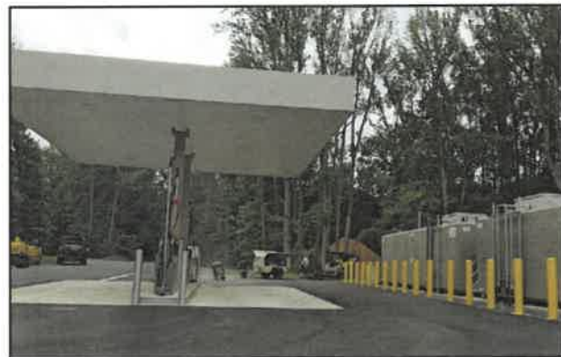
Fuel dispensing island, canopy and ASTs with protective bollards (Under Construction)
