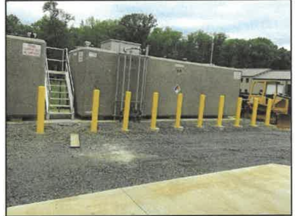
10,000 Gallon AST, fill piping, access stairway and protective bollards (Under construction)
