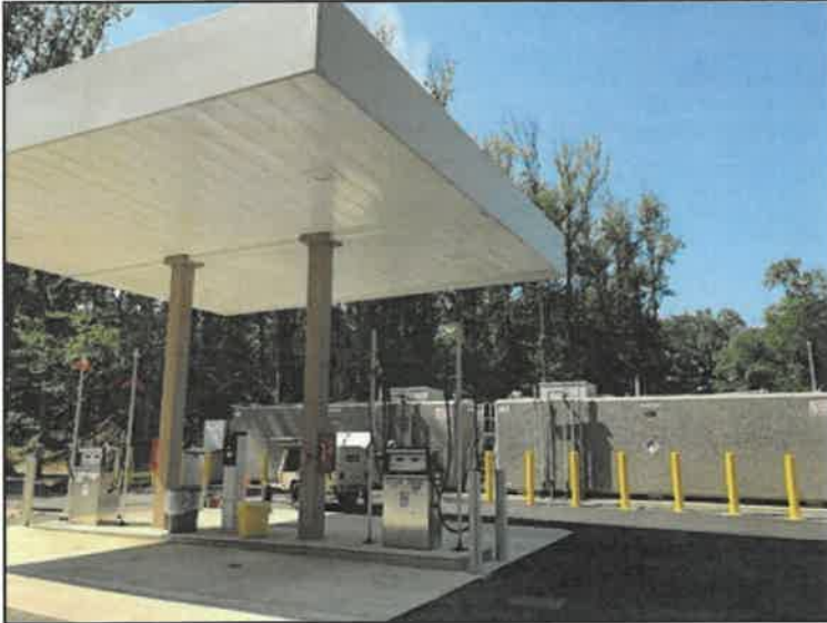
Canopy - Dispenser Island – Above Ground Storage Tanks
